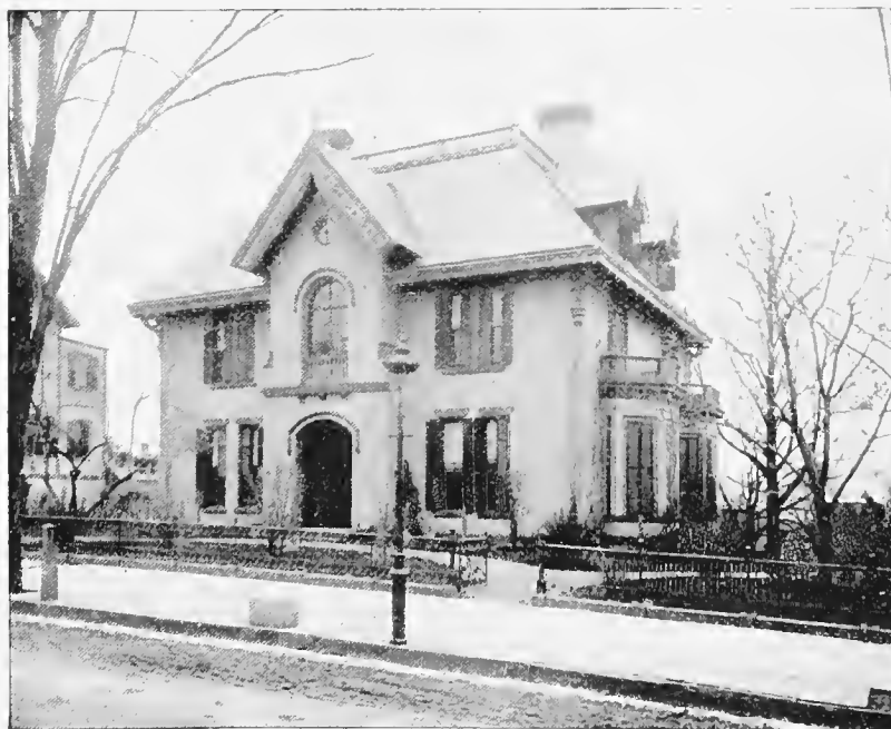
RESIDENCE OF JAMES CHADWICK—182 Grand Street.
